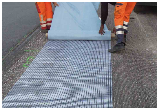
Pic. 2: ADFORS GlasGrid PG application for local repairs
