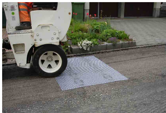
Pic. 3: ADFORS GlasGrid PG installation and adhesive layer activation
