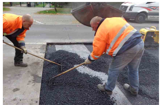
Pic. 9: HMA application over ADFORS GlasGrid PG
