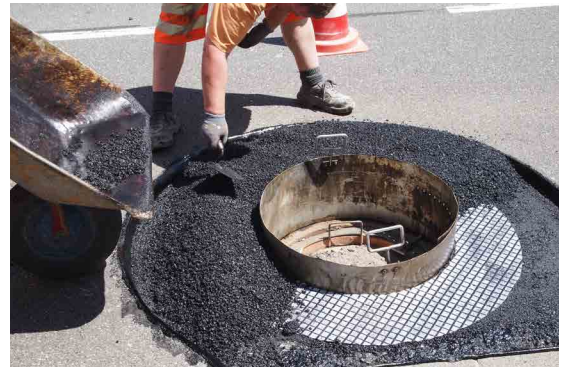
Pic. 8: HMA application over ADFORS GlasGrid PM
