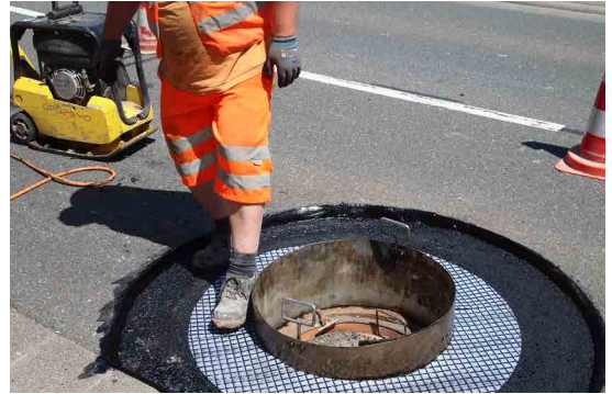
Pic. 4: ADFORS GlasGrid PG installation for manhole repair
