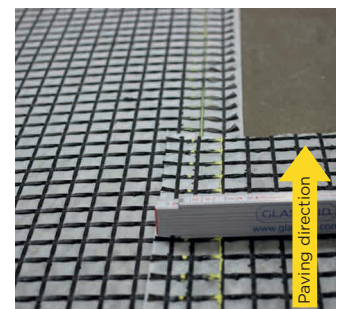
Pic. 6: Longitudinal joints
