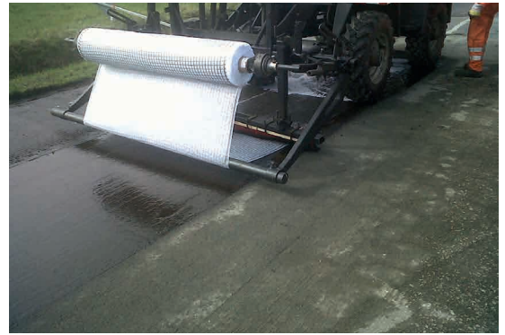
Pic. 4: Fabric Tractor Installation of ADFORS GlasGrid CGL
