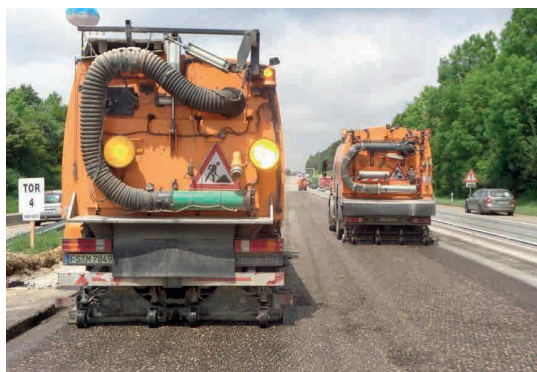
Pic. 1: Ultra High Pressure technology to clean the surface
