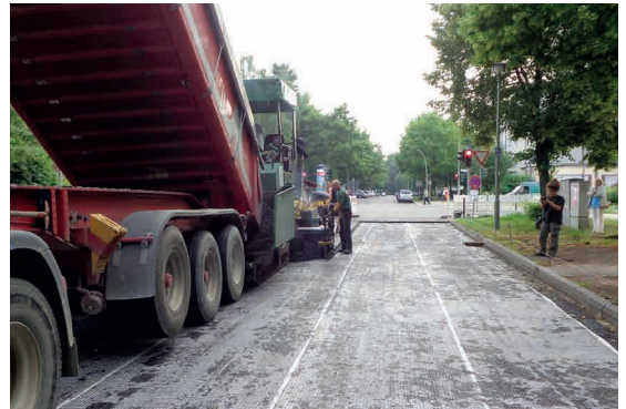
Pic. 9: Pave Overlay
