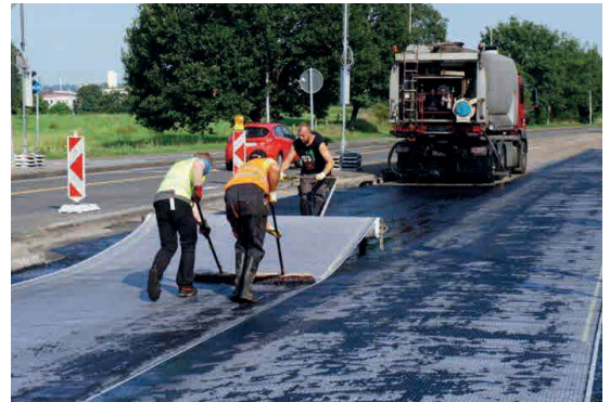
Pic. 5: Manual Installation of ADFORS GlasGrid
