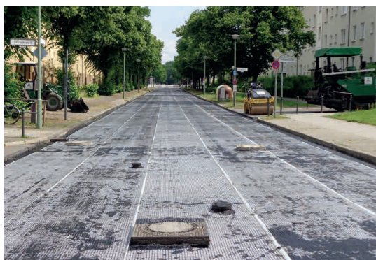
Pic. 2: Typical ADFORS GlasGrid CGL/ CG application on milled surface
