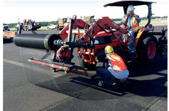
Pic. 3: Fabric Tractor Installation of ADFORS GlasGrid
