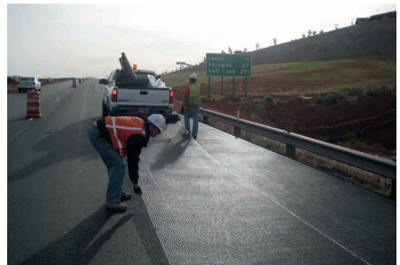
Pic. 4: Manual Installation of ADFORS GlasGrid
