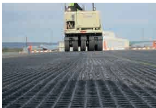
Pic. 2: Typical installation and glue activation on a leveling course
