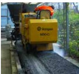
In this test, ADFORS GlasGrid GG200 - 200 kN/m was installed on an existing binder course AC 16 B S and covered with 4cm thick top layer SMA 8 S. The upper part of the binder course including the reinforcement grid were picked up by the milling machine in a single step. No adverse effects were realized and milling depth was not affected.
